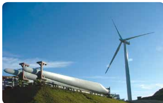
Meridian Energy's West Wind wind farm, to the west of Wellington, was fully commissioned in October 2009. It generated 497 gigawatt hours (GWh) in the year to 30 June 2010.
